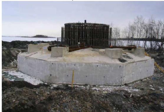
Figure 3: Running the foundation with pile by Rocky Company [6]
