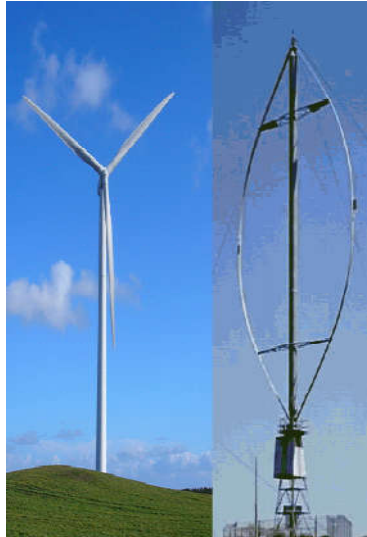
Figure 1: Wind turbine with vertical axis on the right and wind turbine with horizontal axis and on the left [4]
