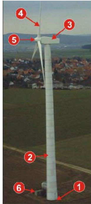
Figure 2: The components of the wind turbine (1 Foundations 2. Rig, 3. System handlers, 4. Rotating screen, 5. Foot of turbine, 6. Converter) [5]
