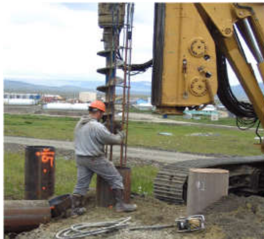
Figure 4: Running the foundation with pile by Rocky Company [6]
