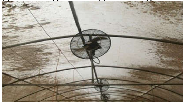
Figure 4; Cooling system fans with spray nozzles mounted at the roof of the house.
